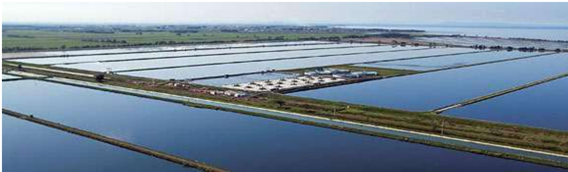
Western Treatment Plant (©Melbourne Water)
