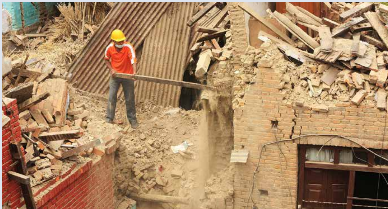
Earthquake damage in Bhaktapur. Photo © UNDP Nepal/Laxmi Prasad Ngakhushi
