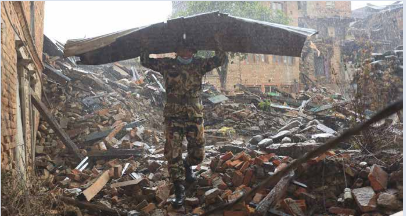
Earthquake damage in Sankhu. Photo © UNDP Nepal/Laxmi Prasad Ngakhushi
