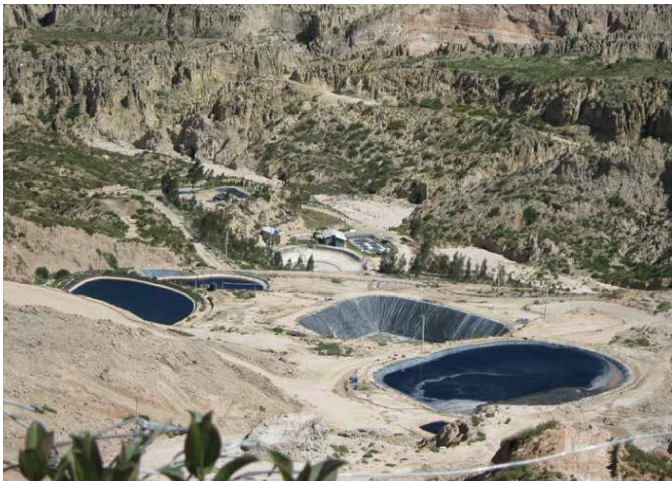
Leachate treatment facilities for a landfill in La Paz, Bolivia. Photo © SWM Department, Ministry of Environment and Water, Bolivia
