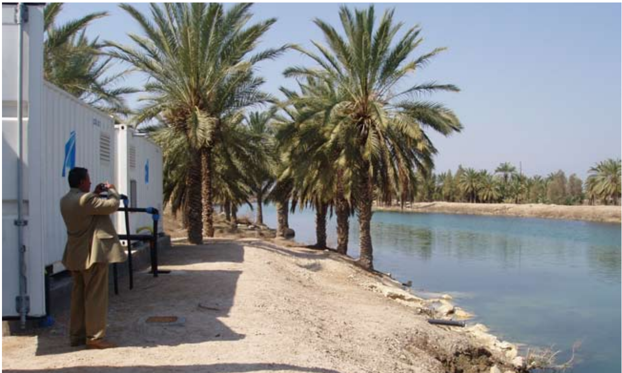
The water plant facility at Al-Jeweber
