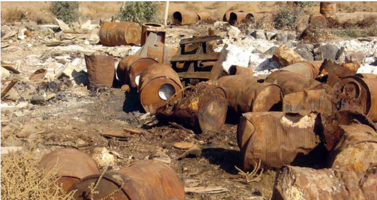
The Al Qadisiya site is unsecured, contains quantities of highly toxic chemicals and has been demolished in an uncontrolled manner, resulting in severe human and environmental hazards
