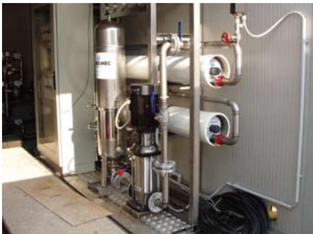
The water plant facility at Al-Kirmashiya
