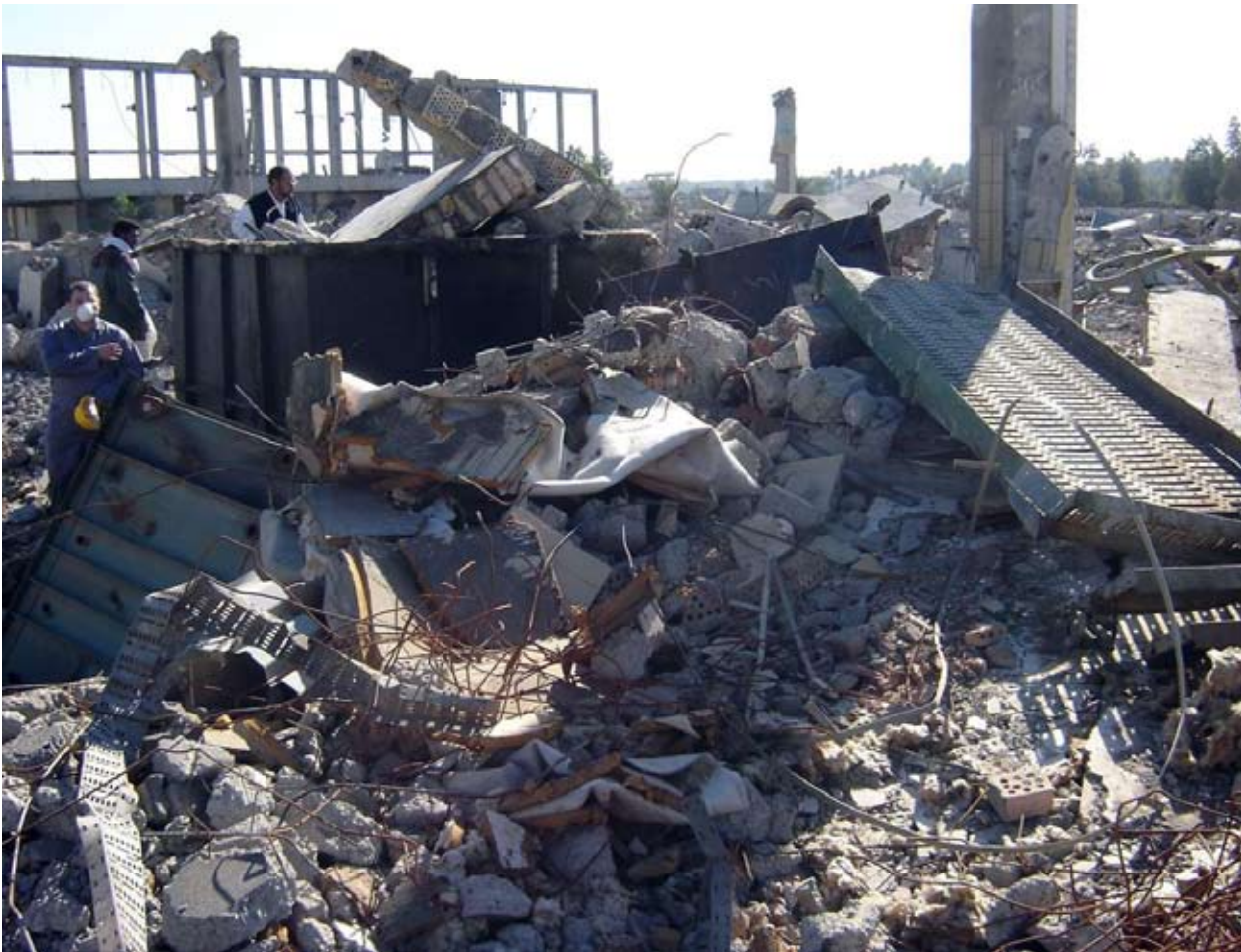
Inspection of a demolition site
