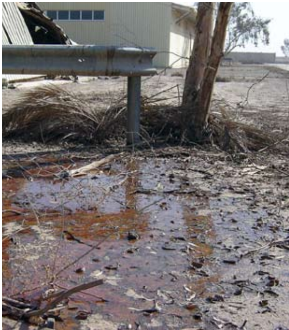
The site of Khan Dhari used to be the Iraq central refinery chemicals warehouse facility. It now represents a moderate risk to the health of site workers, and as such is unfit for normal use
