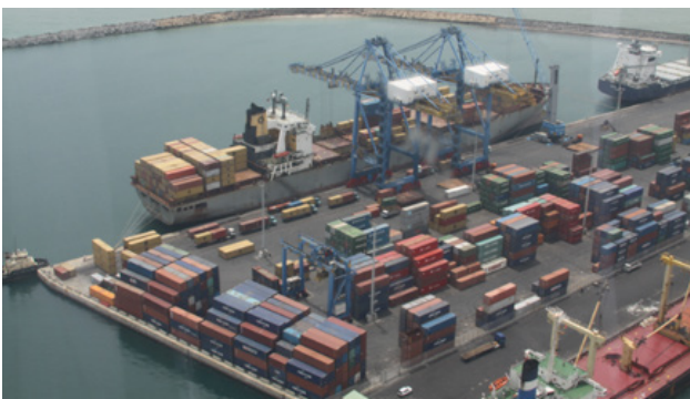
MPS Dedicated container terminal
