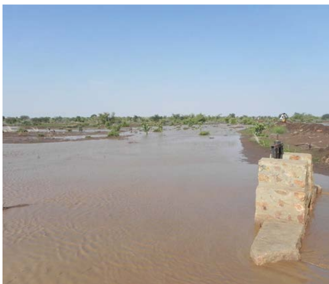
Large areas of wadi land covered by water retained by rehabilitated Eware structure and released for irrigation
