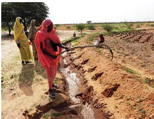
Construction of small earth terraces to reduce gully erosion as part of a community awareness raising campaign
