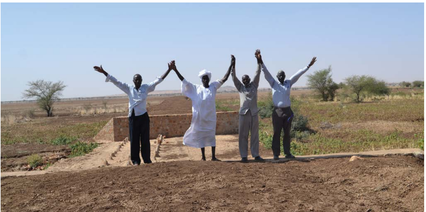
New concrete spillway constructed (30 m length; 6m width)
