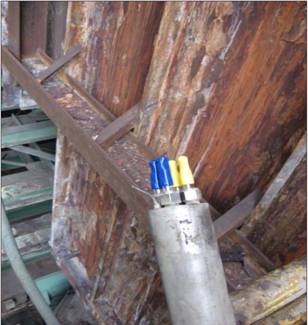
Figure I-5: Sample probe with end caps installed
