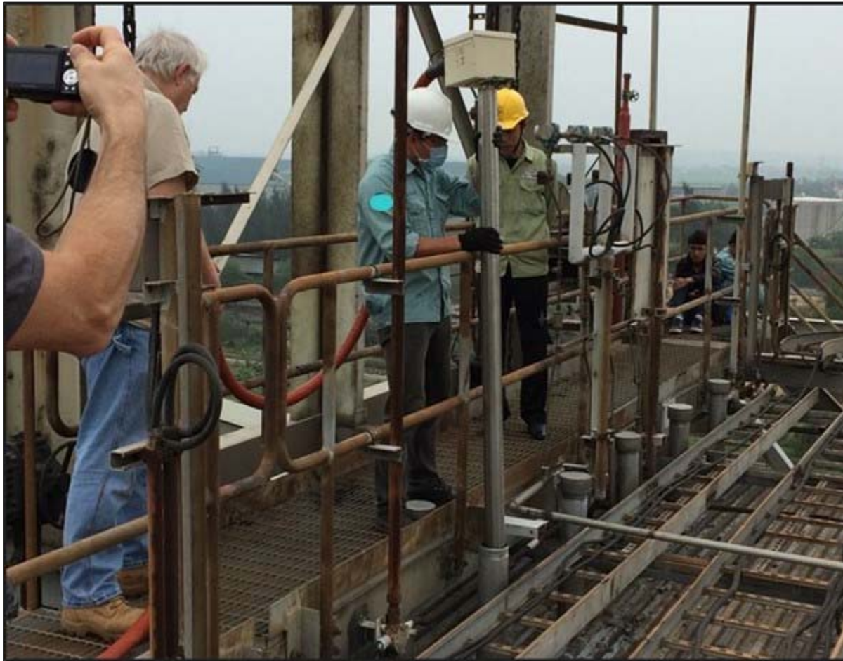
Figure I-6: Sample probe insertion into stack
