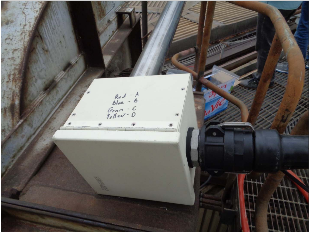
Figure I-4: Heated sample line strain relief attachment to heated filter box
