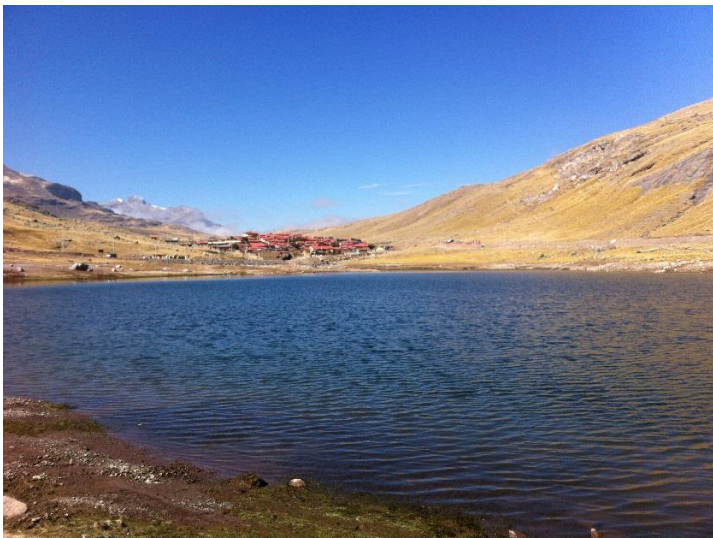
Tanta: Water reservoir
