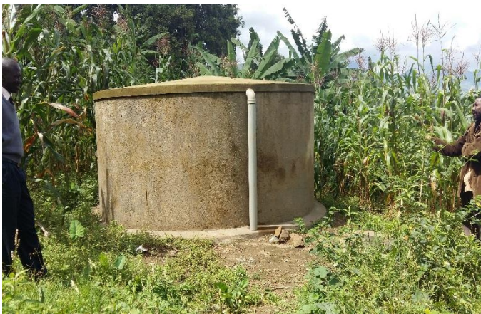
Storage tank for gravity water scheme in Sironko District
