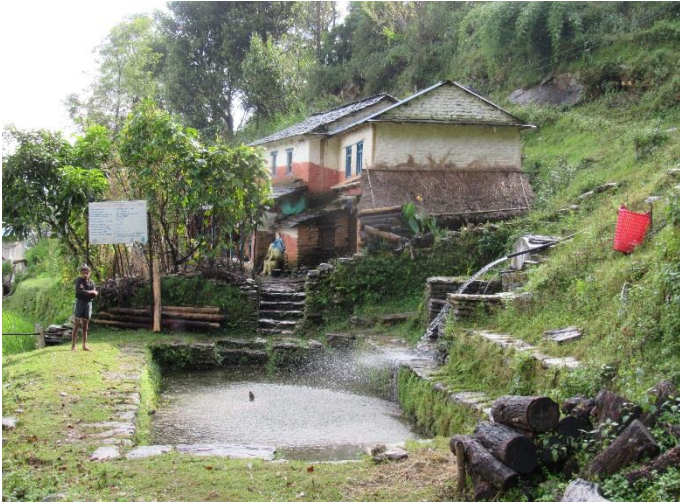
Panchase: River bank protection using bio-engineering technology
