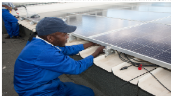
Installation of Solar Panels in Namibia UN House, 2017
