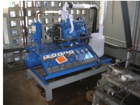
R404A compound compression unit of a blast freezer for meat products (cycle -36 / +32 °C)
