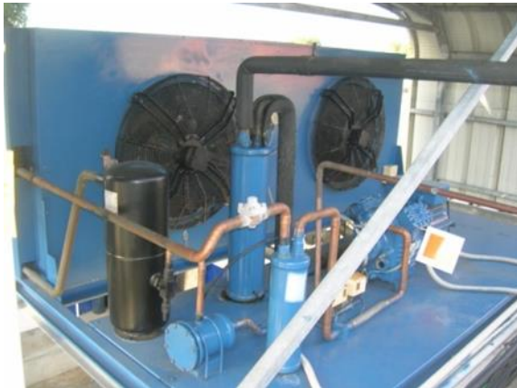
R134a condensing unit for the process of a vegetable work area (cycle -3 / +32 °C)
