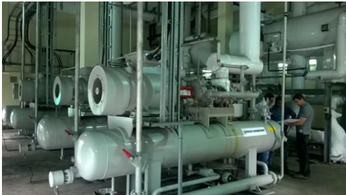
R404A screw compressor and separation receiver for a large -25°C warehouse (cycle -35 / +32 °C)
