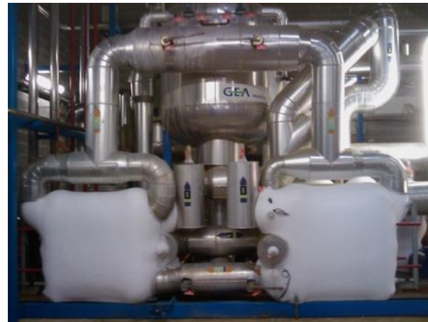
Ice water production (-7 / -2°C) with plate heat exchangers fed by thermosiphon on a R717 separation receiver (cycle -15 / +32 °C)
