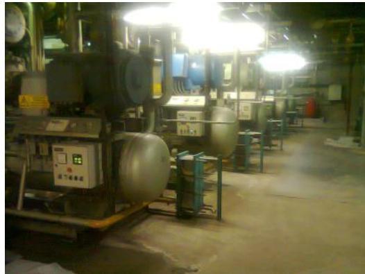
A typical industrial machinery room with liquid / vapor separation receiver (on the left) and screw compressors (on the right)
