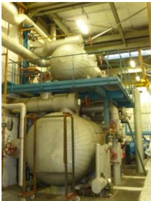
A typical industrial machinery room with liquid / vapor separation receiver (on the left) and screw compressors (on the right)
