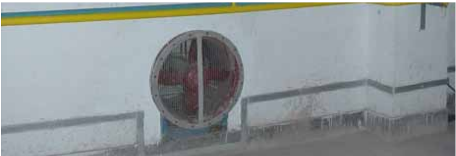
Figure 30. Local air exhaust device
