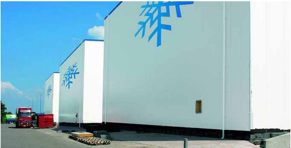
Figure 27. PU building thermal insulation panel are widely used in assembled cold storages
