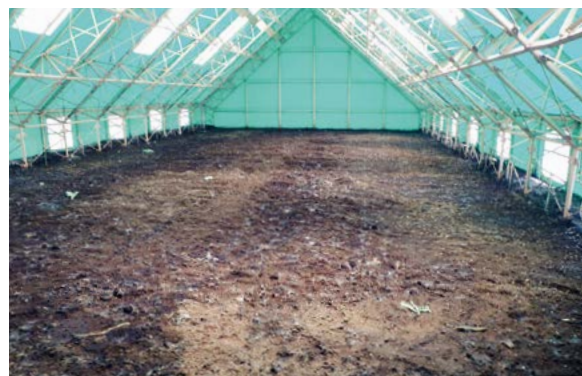
Fig. 30 Soil for deodorising in Nagai City, Japan
