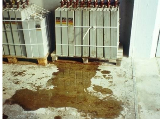
Picture 85: Bad example II (no tip trays)
