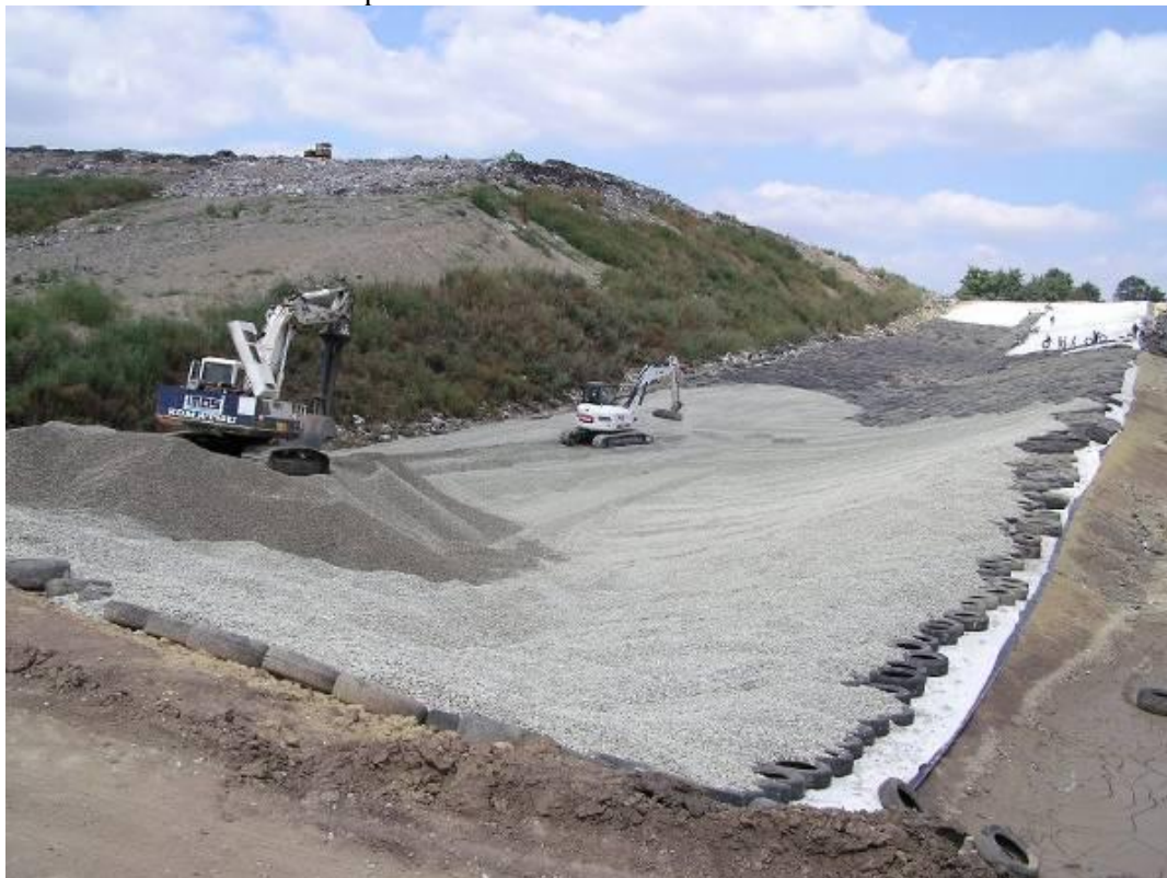
Fig. 34: Artificial geological barrier for landfill
