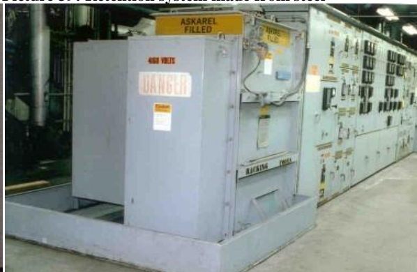
Picture 39: Retention system made from steel
