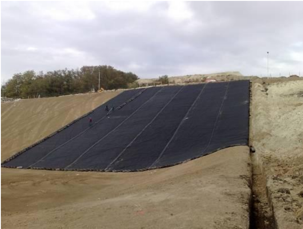
Fig. 35: Artificial barrier using HDPE foil for landfill
