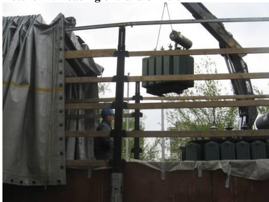
Picture 71: Loading of transformers
