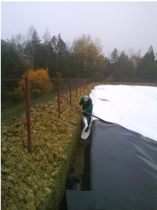
Fig. 36: Foundation of landfill
