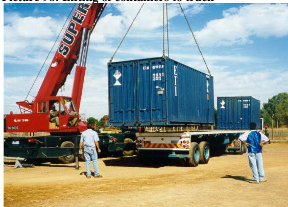
Picture 98: Lifting of containers to truck
