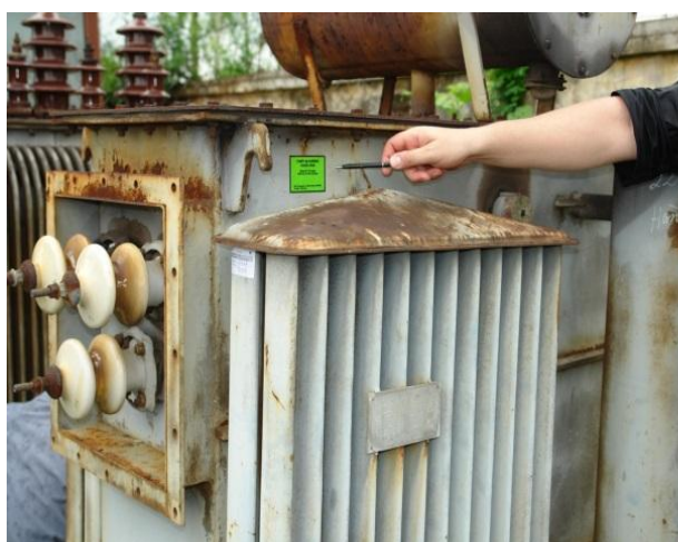
Picture 12: Affix labels while sampling and later final one
