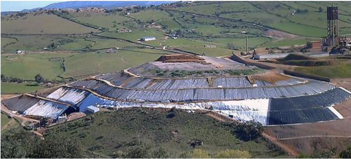
CERCO DE SAN TEODORO SLAG HEAP MARCH 2007
