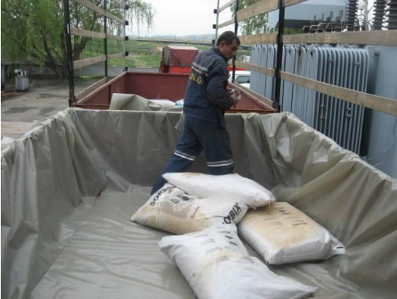
Picture 69: Preparation: transportation of PCB transformer
