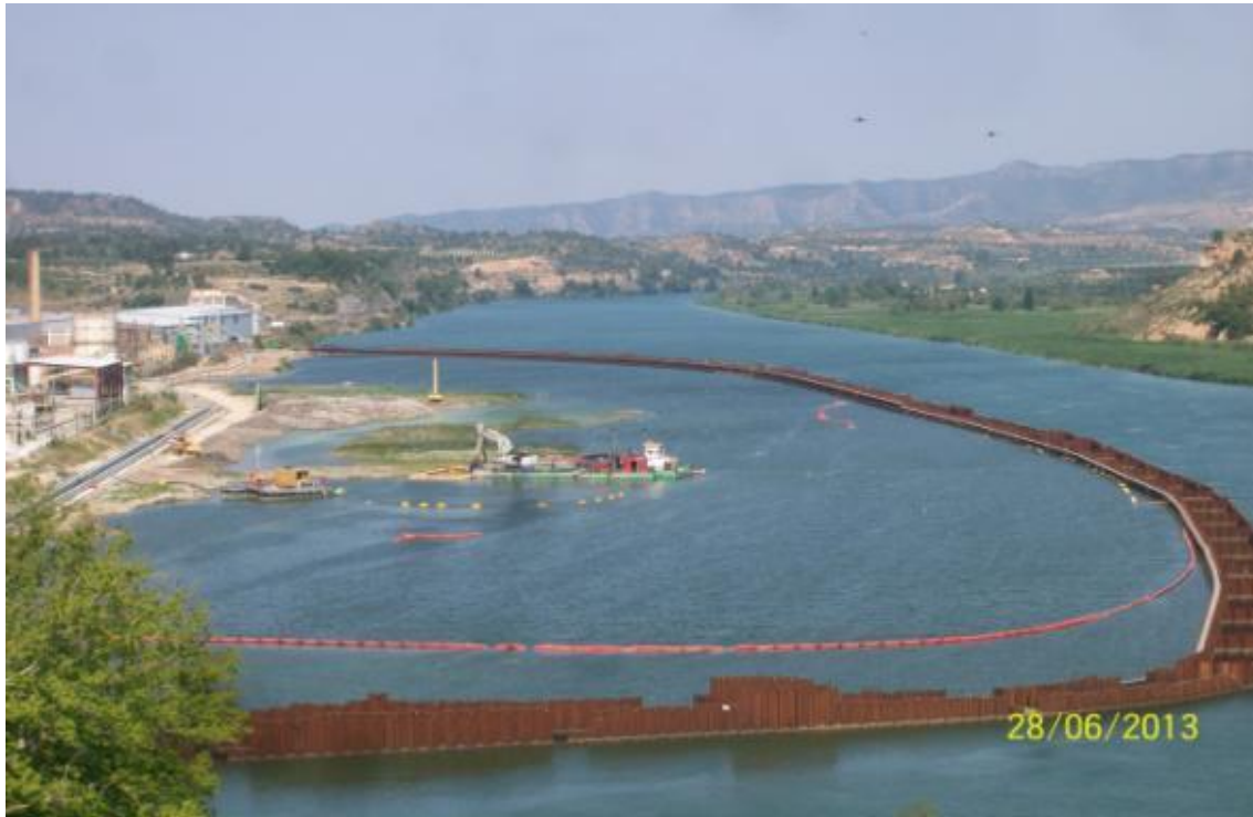
Dredging activities inside the sheet piling
