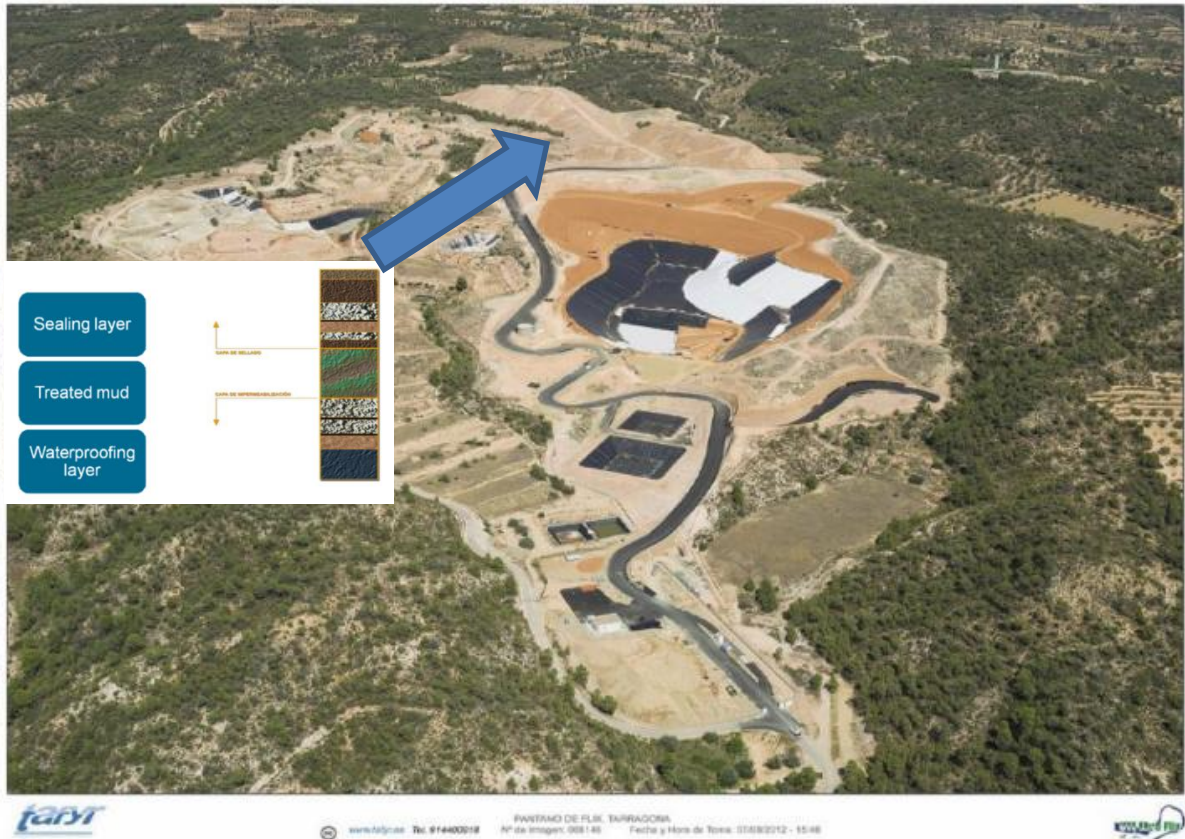
Conditioning works in the “Racó de la Pubilla” Landfill
