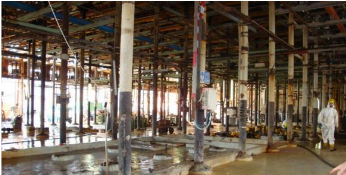
Floor of cell room regularly washed down
