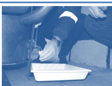
Place drip tray under drain tap, wearing gloves and goggles
