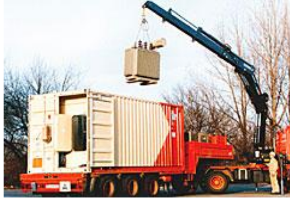
Picture 100: Loading of transformers
