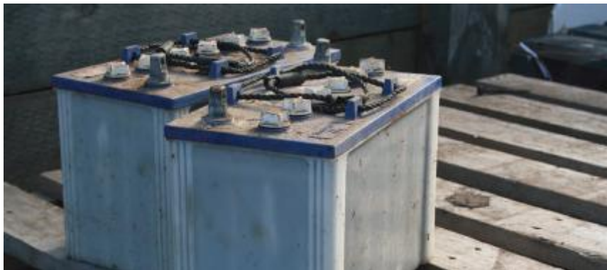
Fig. 46: Examples of bad used lead batteries management
