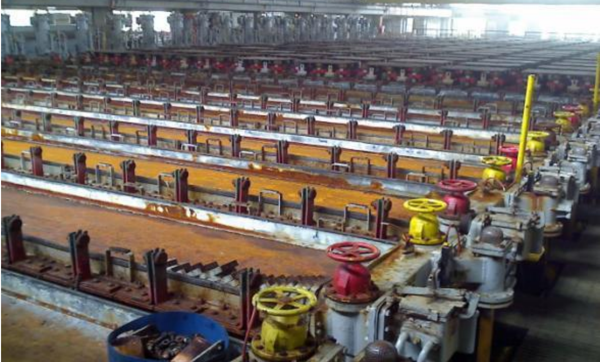
First stage of operations
