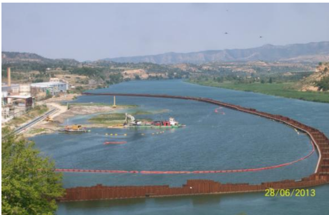
Dredging activities inside the sheet piling
