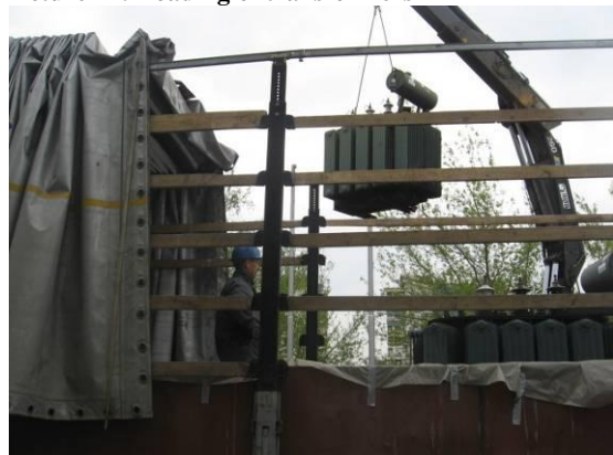
Picture 71: Loading of transformers
