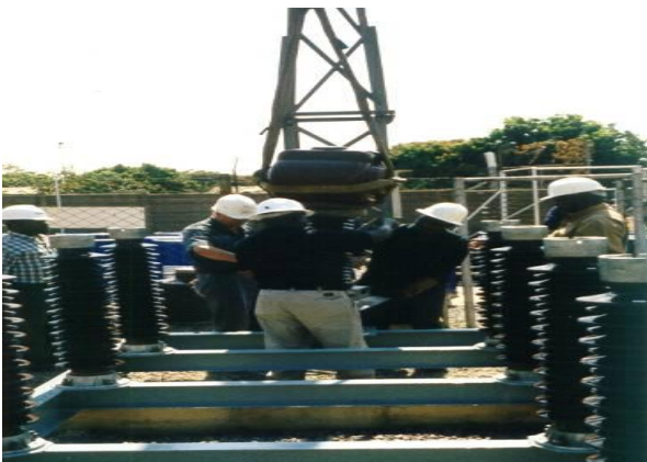
Picture 55: Dismantling of capacitor battery
