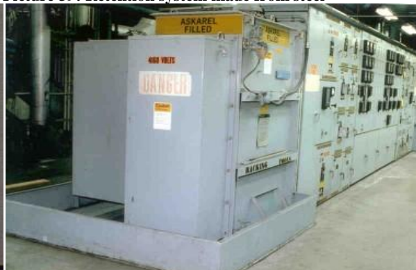
Picture 39: Retention system made from steel
