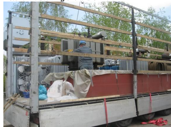
Picture 72: Stowing of transformers
