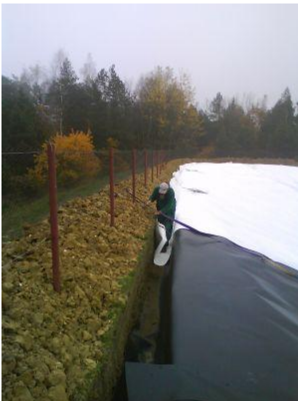
Fig. 36: Foundation of landfill
