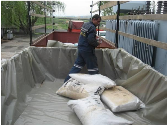
Picture 69: Preparation: transportation of PCB transformer
