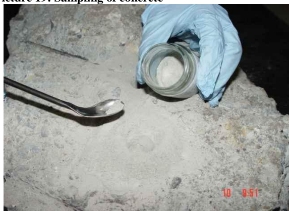
Picture 19: Sampling of concrete
