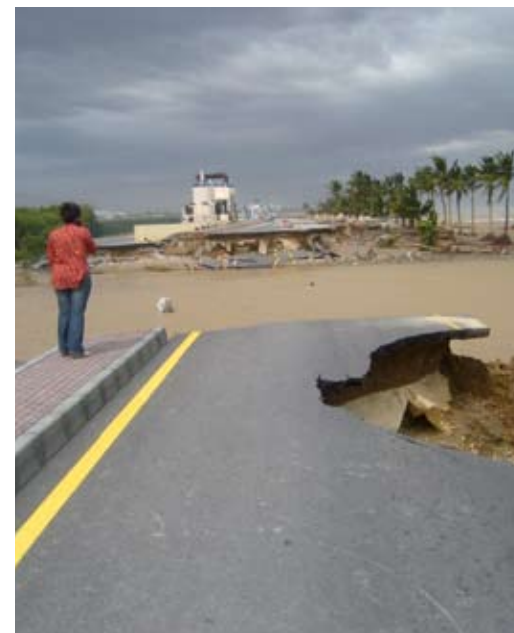
Cyclone Gonu left a path of destruction—flooding streets, downing power lines, damaging water supplies, and undermining coastal infrastructure.
