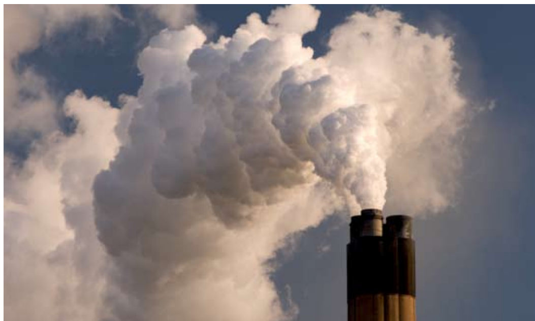
Emissions from the Eggborough coal-fired power station in Yorkshire, UK. The relentless growth of coal-dependant energy production—China plans to build 544 new coal-fired stations in the next decade—presents a serious challenge to avoiding climate change.
