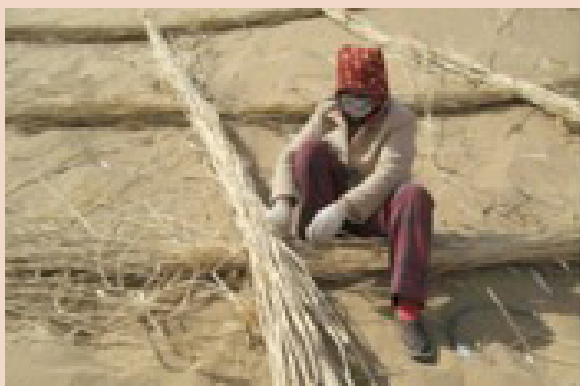
Initial stabilization of sand dunes using checkerboards
