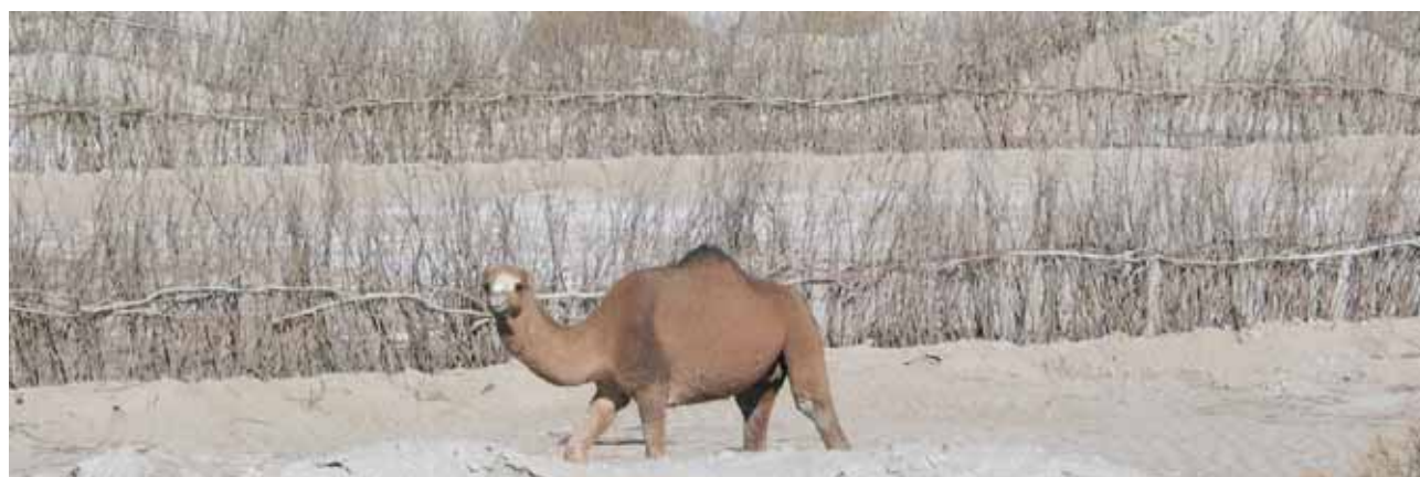
Hundreds of kilometres of windbreakers were constructed in the Sistan Basin lakebeds to trap the wind-blown sand
