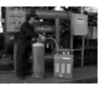
A Navy service technician recovering refrigerants from a system during regular maintenance. Training technicans in good maintenance procedures to avoid accidental releases, prevent refrigerant leaks, and recover and recycle refrigerants can reduce operating costs, increase refrigeration system efficiency, and protect our environment at the same time.
