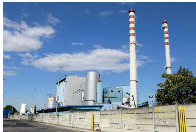
Waste to energy plant in Lombardy, Italy
