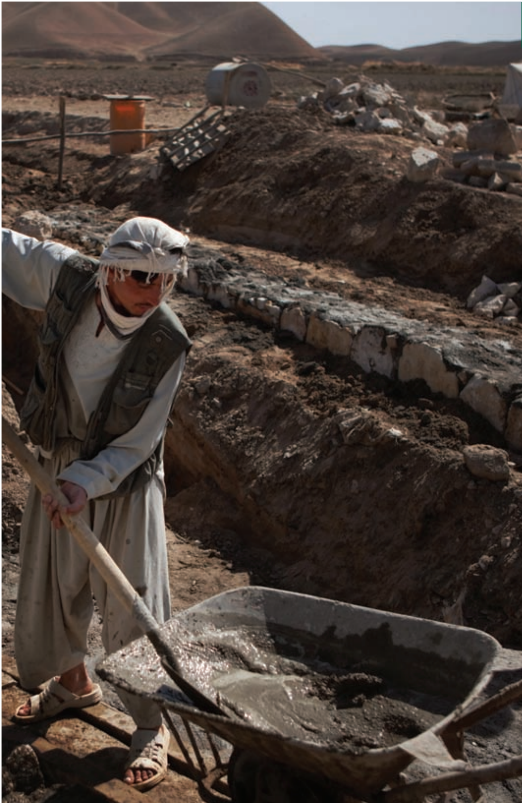
Workmen constructing an irrigation channel, Afghanistan.
