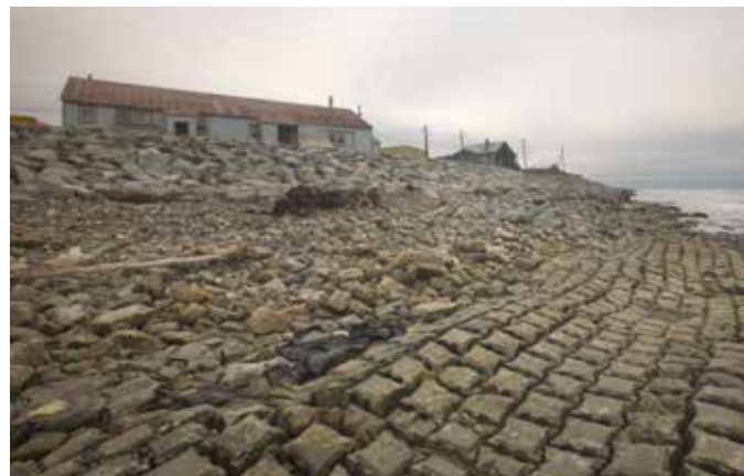
Protection against severe erosion of the coastline in Shishmaref, Alaska, United States. The reduced period in which there is sea ice has made sandy sediments more vulnerable to erosion. Credit: Lawrence Hislop
