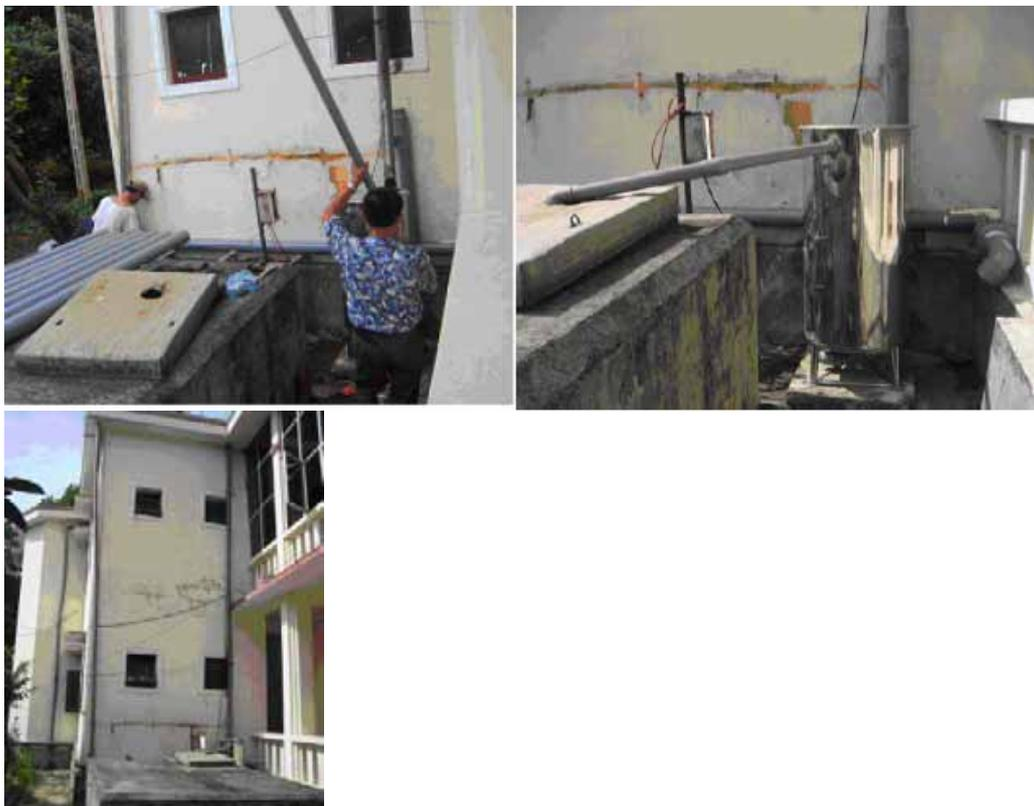
Picture 3 Installation of rainwater harvesting system at the company
