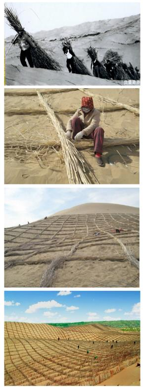
**Figure 4.4.** Sand barrier technology using a grid pattern of bundled Salix (willow) stems, crop straw and other materials.
