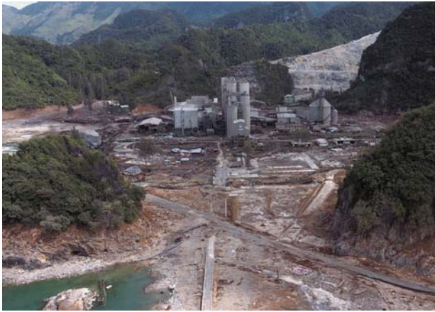
Cement factory along the tsunami-battered coast of Banda Aceh.
