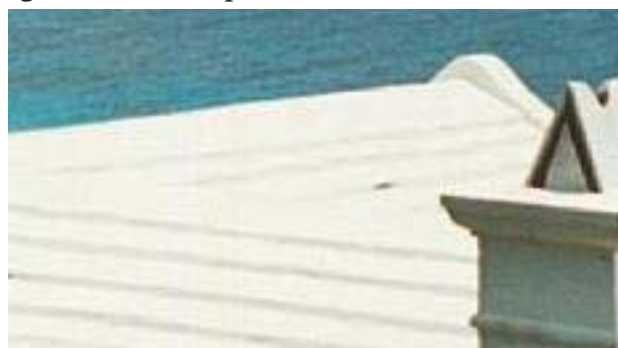
Figure 3.3 Rooftop water catchment
