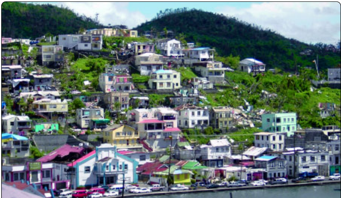
Hurricane damage in Grenada
