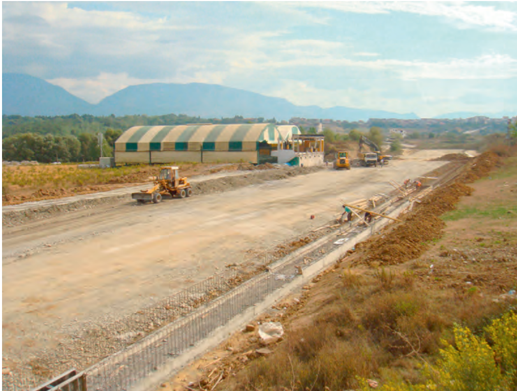
Photo 2.1: Highway construction in Tirana
