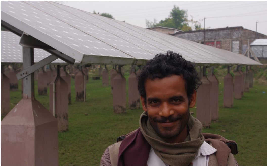
A mini-grid operator standing in front of a 120 kW PV installation on Sagar Island, India photo credit: Juan Pablo Carvallo Bodelon
