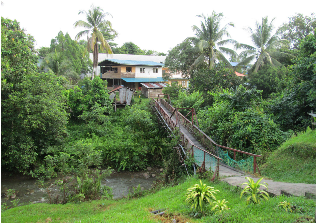
A small community in Borneo with substantial unexploited hydropower potential
