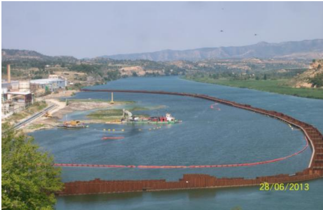
Dredging activities inside the sheet piling
