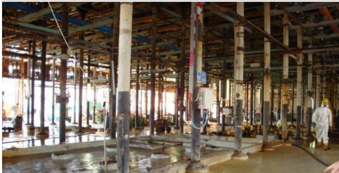
Floor of cell room regularly washed down
