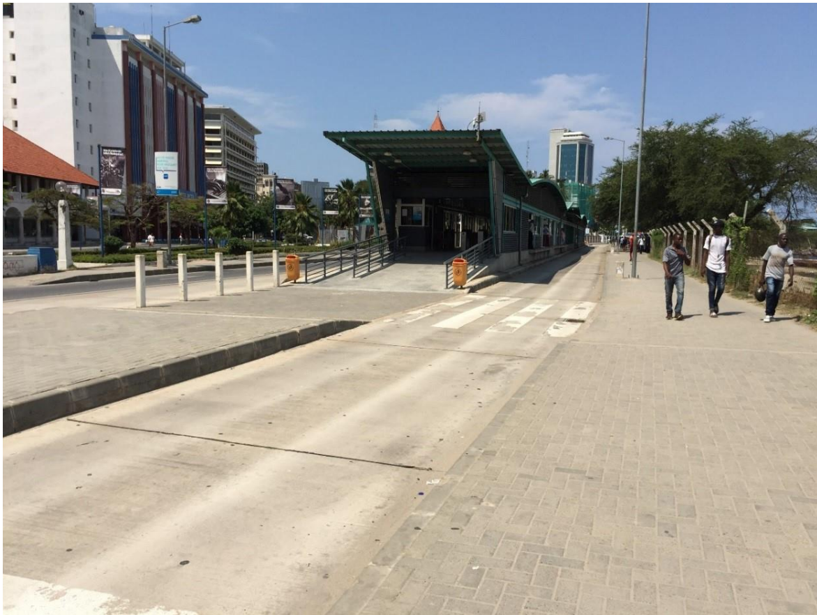
Picture 2: Posta BRT Station near Kivkoni Ferry Terminal along Mongoro trunk line in Dar es Salaam
