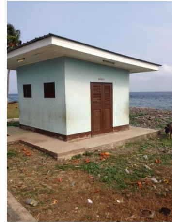
Figure 12: Public toilet constructed at beach, STP, Jul 2018
