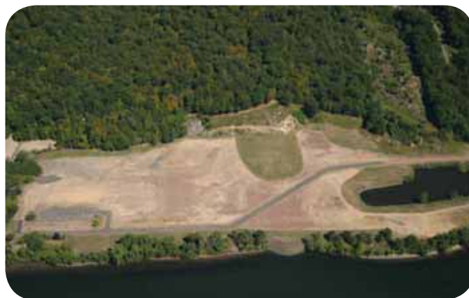
Figure 11: The Connecticut Yankee nuclear power plant was successfully decommissioned and the site restored to a greenfield. The pictures show progress over time at the start (June 2003), during operations (January 2006) and after decommissioning was completed (September 2007).
