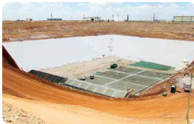
A typical disposal method for low level radioactive waste is burial underground. Care needs to be taken that water does not transport radioactive isotopes beyond the burial site. Credit: US NRC
