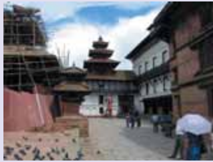
Kathmandu Durbar Square with Jagannath Temple being renovated
