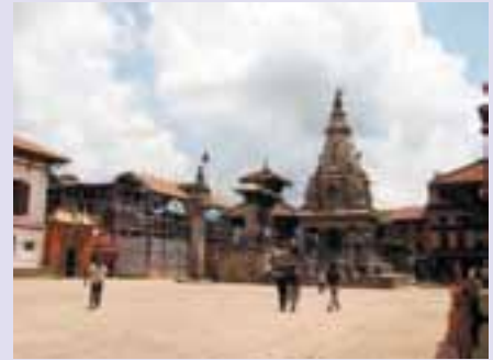
Bhaktapur Durbar Square with the fifty-five windows' palace being renovated
