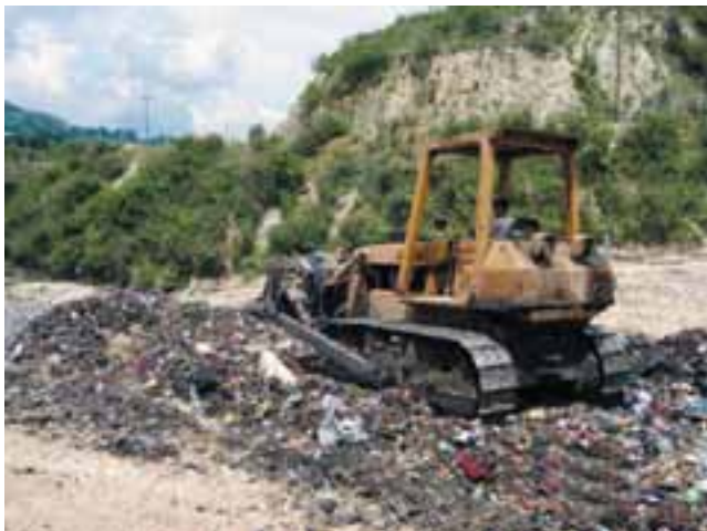
Sisdole compaction
