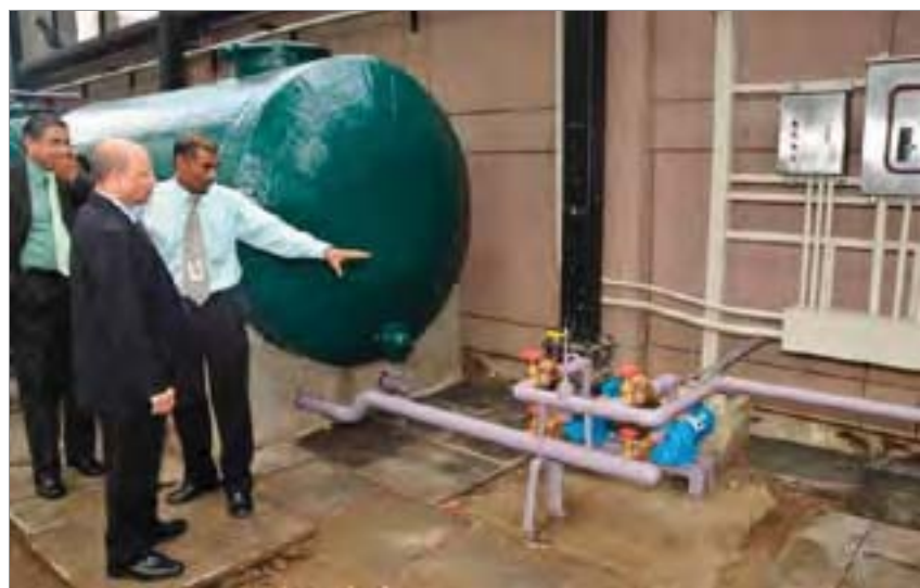
Demonstrating the new rainwater harvesting system to Vice-President Bindu N. Lohani
