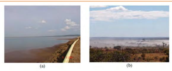
Tailing impoundment (a) – wet part; (b) dry part providing dust fallout affecting plant leaves (Photos courtesy of Nyambe, 2005)
