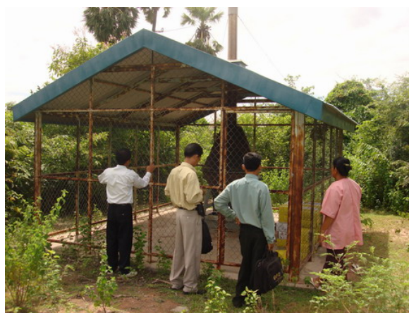
A type of medical waste incineration facilities operating in Cambodia
