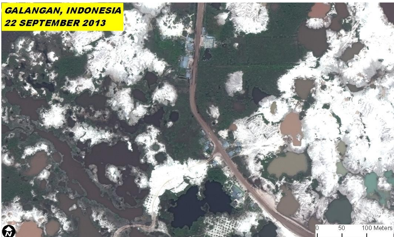
Figure 8: Galangan (22 September 2013) – A small settlement along the main road in northwestern Galangan that is surrounded by open mine pits.
