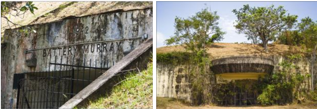
Bunkers located in the Special Economic Area, Panama Pacifico
