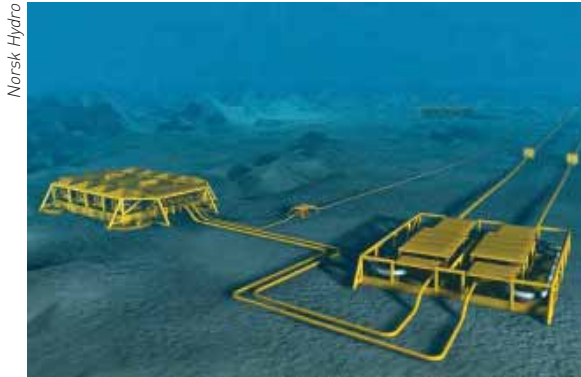
Artist's view of the Ormen Lange field subsea installations off Norway. The templates will be at depths of around 800 – 1 100 metres.
