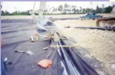
Constructing sanitary landfill in the Caribbean
