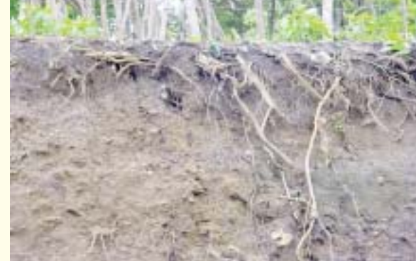
Some land-use practices such as cutting slopes have resulted in massive soil erosion...
