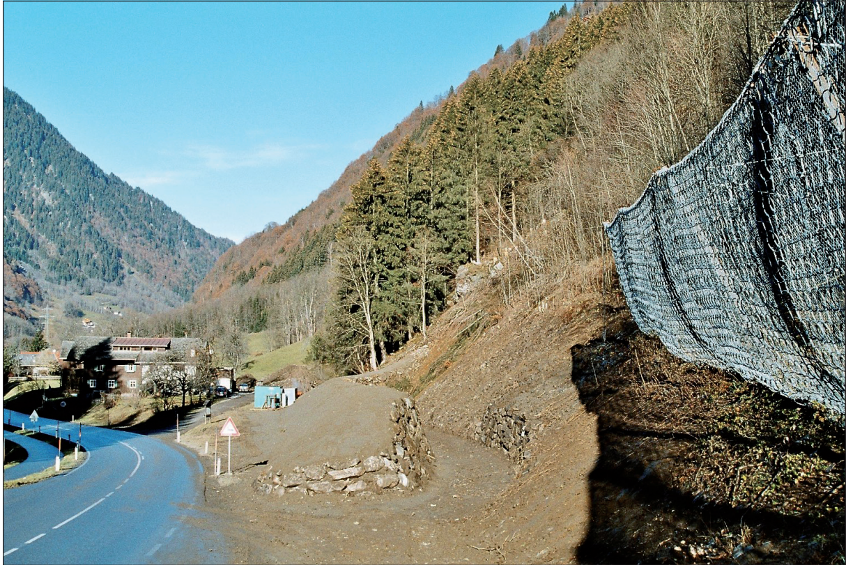
Figure 3. An Austrian mountain road threatened by rock fall with three different protection measures commonly used in the Alps: a rock fall net, a rock fall dam and a protection forest Credit: L. Dorren, 2004
