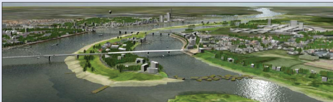
Figure 7. Computer rendering of the Lent-Nijmegen project site after implementation of the measures (Kingdom of the Netherlands, 2011)
