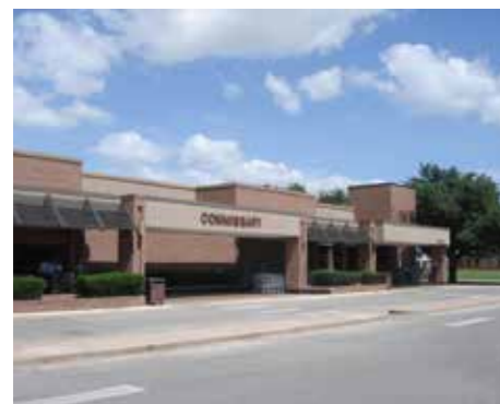
Fig. 1 Outside the Lackland commissary. Photo courtesy of CTA Architect Engineers.
