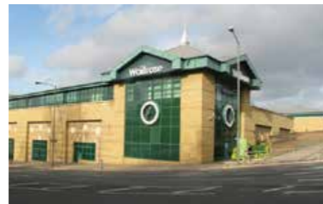
Fig. 1 Photo of the Waitrose store, Bromley South
