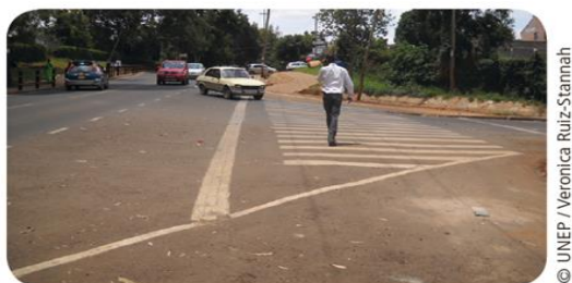
Figure 30: Large turning radius of intersection enlarge the distance for pedestrian and cyclist crossings, and facilitate cars turning at high speed.
