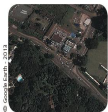
Figure 16: Aerial image of the Limuru Junction after the upgrade in 2013
