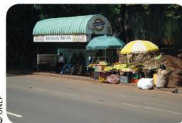
Figure 20: Bus shelter and bay on Limuru Road, direction to Ruaka
