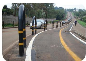
Figure 25: Bollard separator without kerb
