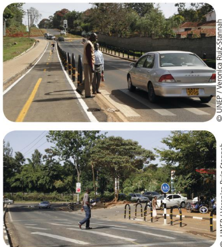
Figure 29: Raised zebra crossing vs. painted-only crossing. The second ones do not act as traffic calming devices.
