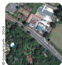
Figure 15: Aerial image of the Limuru Junction before the upgrade in 2010
