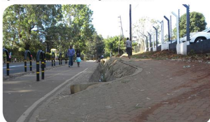
Figure 32: Detour and different grade of sidewalk
