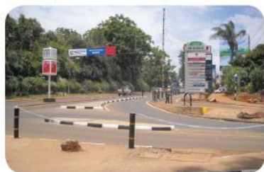
Figure 18: Slip-lanes with medians to facilitate pedestrian crossing
