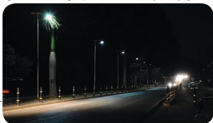
Figure 31: Solar-led lights provide environmentally friendly light
