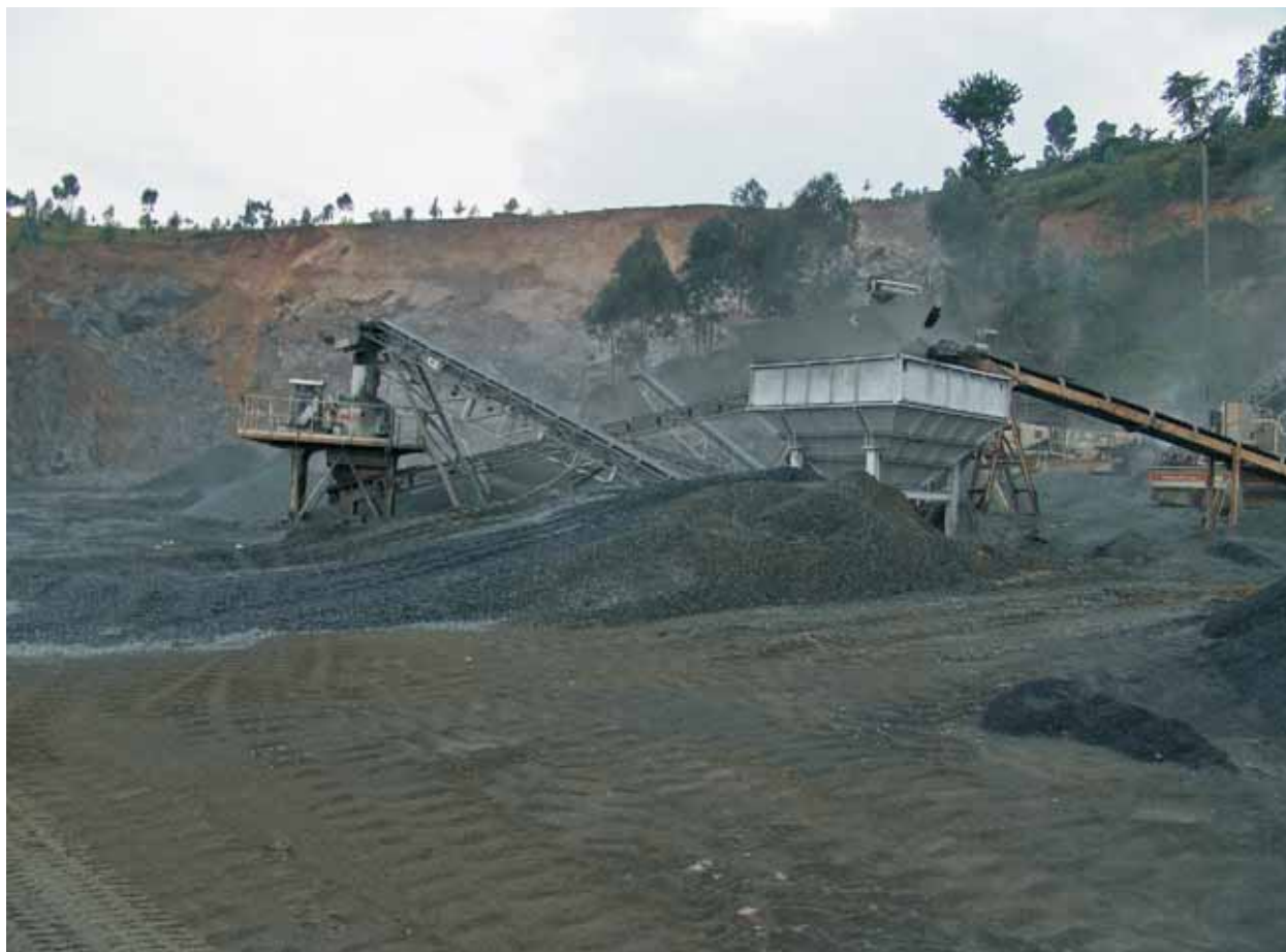
Large-scale quarrying for road materials
