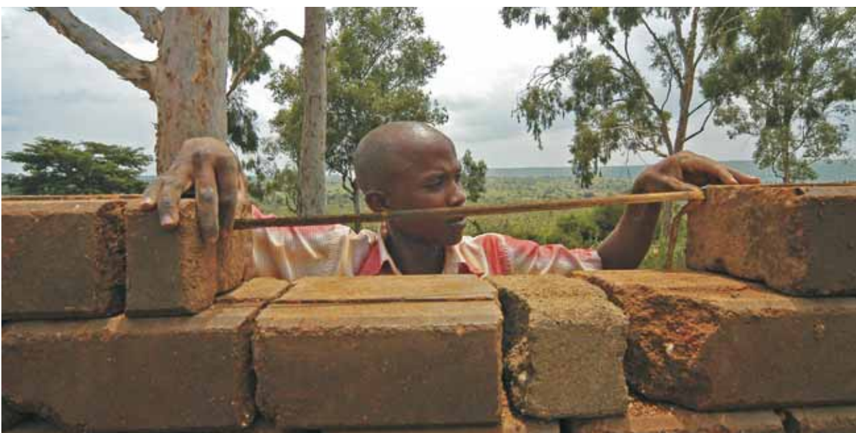
Building houses in Bukora resettlement site for Rwandan returnees from Tanzania
