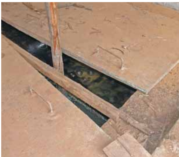
Industrial wastewater is drained from holding tanks and its untreated contents disposed of at the Nyanza dumpsite
