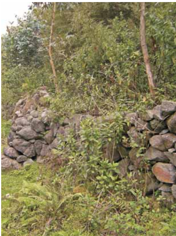
The Volcanoes National Park is delineated by a simple rock wall that serves to curtail raiding of crops by wildlife, particularly buffalos, as well as inhibit encroachment by farmers
