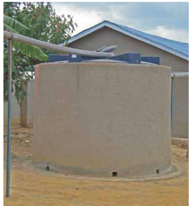
Rainwater harvesting helps alleviate water shortages in drought prone areas such as in Rwimikoni village, Bugesera District
