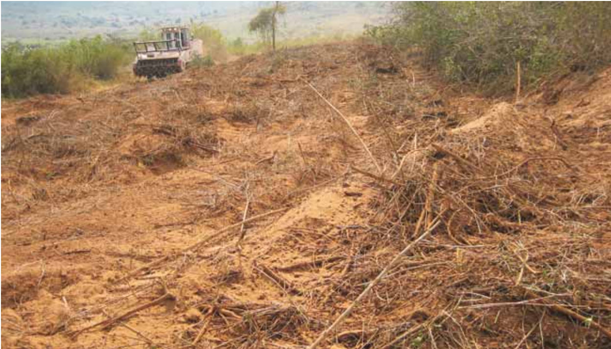
Legacy of the 1990-1994 conflict, the Kanombe minefield outside Kigali required mechanical demining due to thick vegetation and difficult terrain
