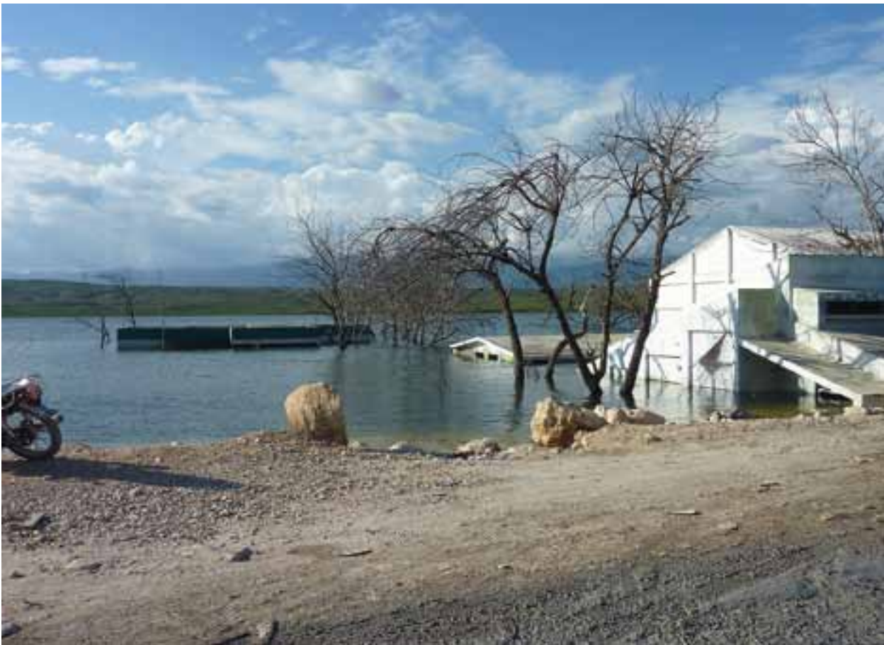
Investments that have been made in the last five years to provide Haiti with modern custom and immigration facilities along the main road connecting the two countries are now inoperative and partially submerged as a result of the rising water levels in Lake Azuei.
