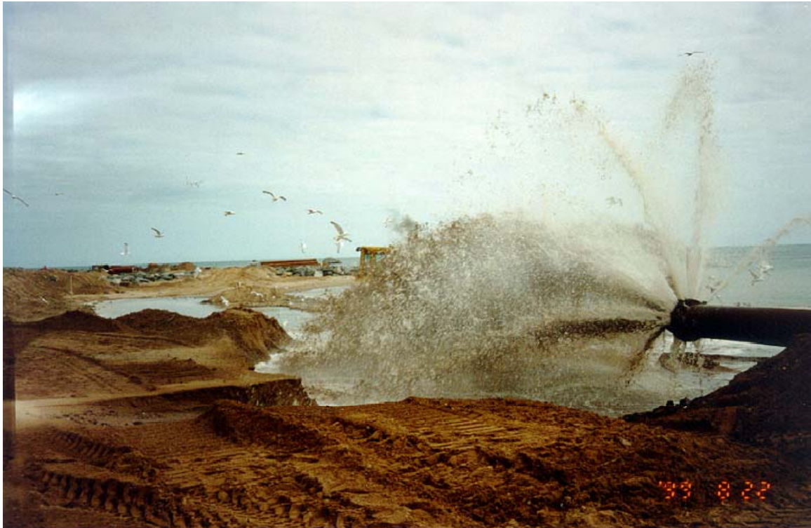
Figure 4.3 Artificial Nourishment of beaches
