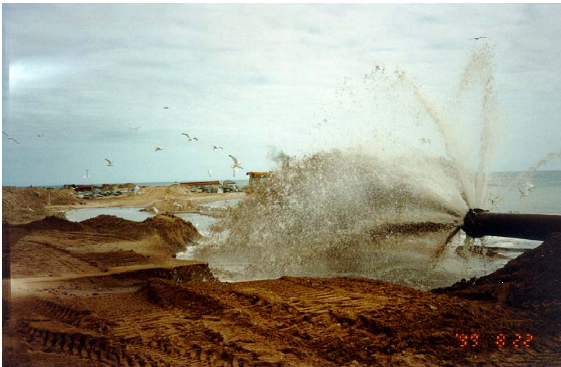
Figure 2.6 Artificial Nourishment of beaches
