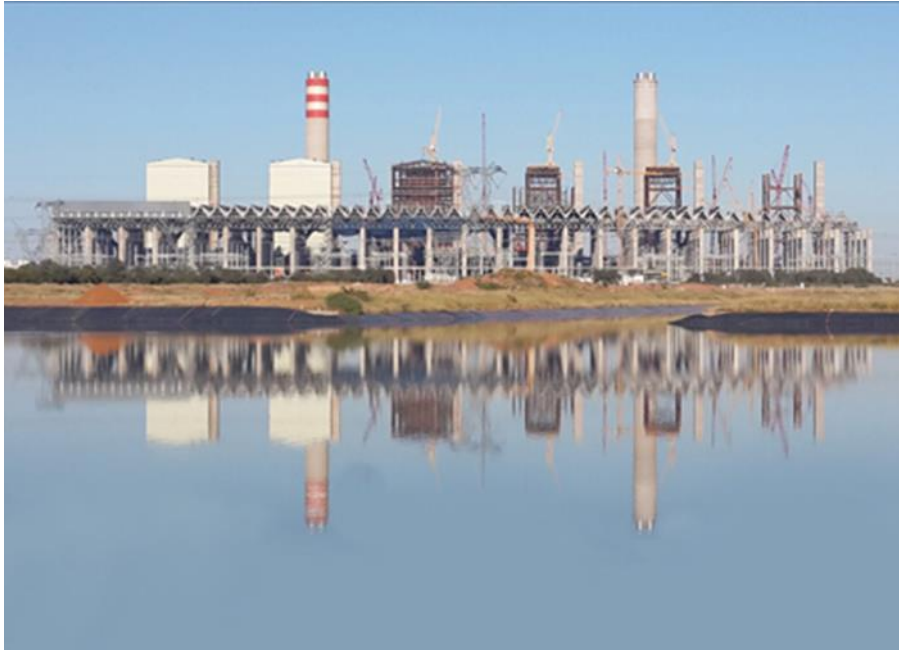
Figure 4 Medupi -Eskom’s Supercritical, dry-cooled plant (Robb, 2017)
