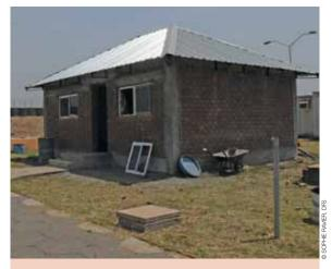
2) Alternative construction materials to reduce deforestation pressure: To reduce deforestation pressure and water consumption, UN Mission in Darfur (UNAMID) replaced traditional building bricks with compressed soil blocks. This led to a 30 percent reduction in water use and 100 percent reduction in fuelwood consumption. The bricks were subsequently adopted by the United Nations Mission in South Sudan (UNMISS) as well as other humanitarian actors working in the region.
