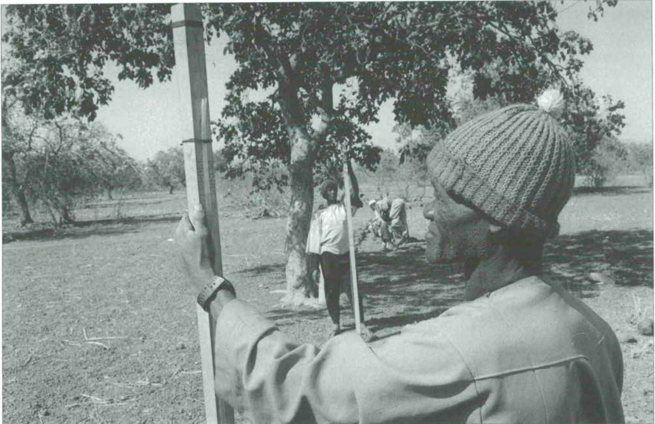
Burkina Faso: measuring level contours to build stone lines and prevent soil erosion
