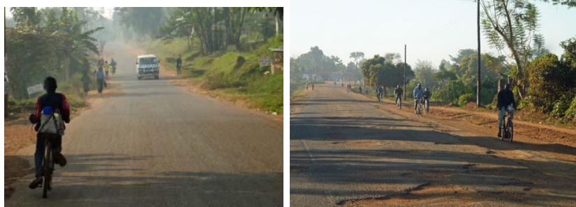
Left: Sandy runoff encroaching a road. Right: Off-road pedestrian footway formed to avoid dangerous vehicles
